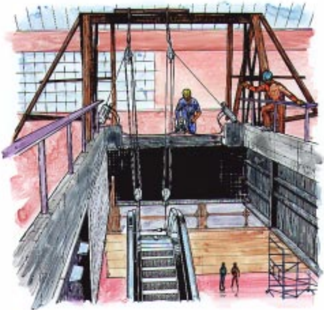
Fig. 27 - Installation of mechanical escalator (TU-16H)
